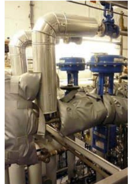
Steam valve insulation
