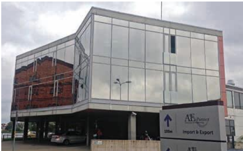
Outside facade covered with a solar reflective control film
